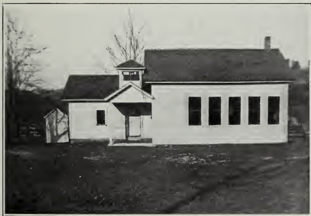
A one-room rural school before and after repairs were made
